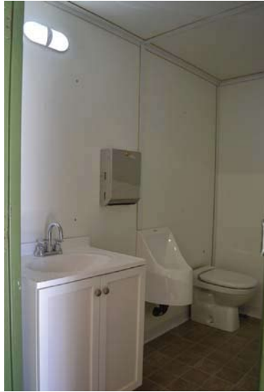
Restroom with Vacuum Toilet, Waterless Urinal, and Sink
